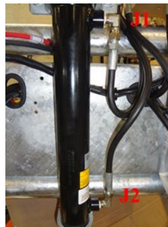
Jack hose installation (18” Hoses)
